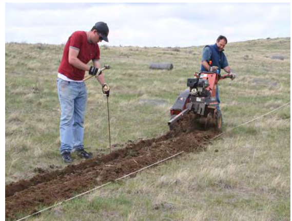
Figure 10: Using a Self-Propelled Trencher to Install a Barrier Fence
