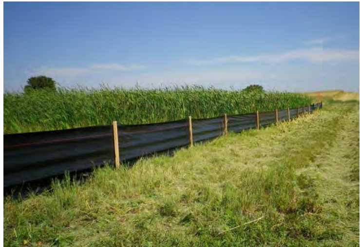
Figure 9: Barrier Fence Constructed of Geotextile Fabric (Photo by Jamie Sparrow, Golder Associates Ltd.)
