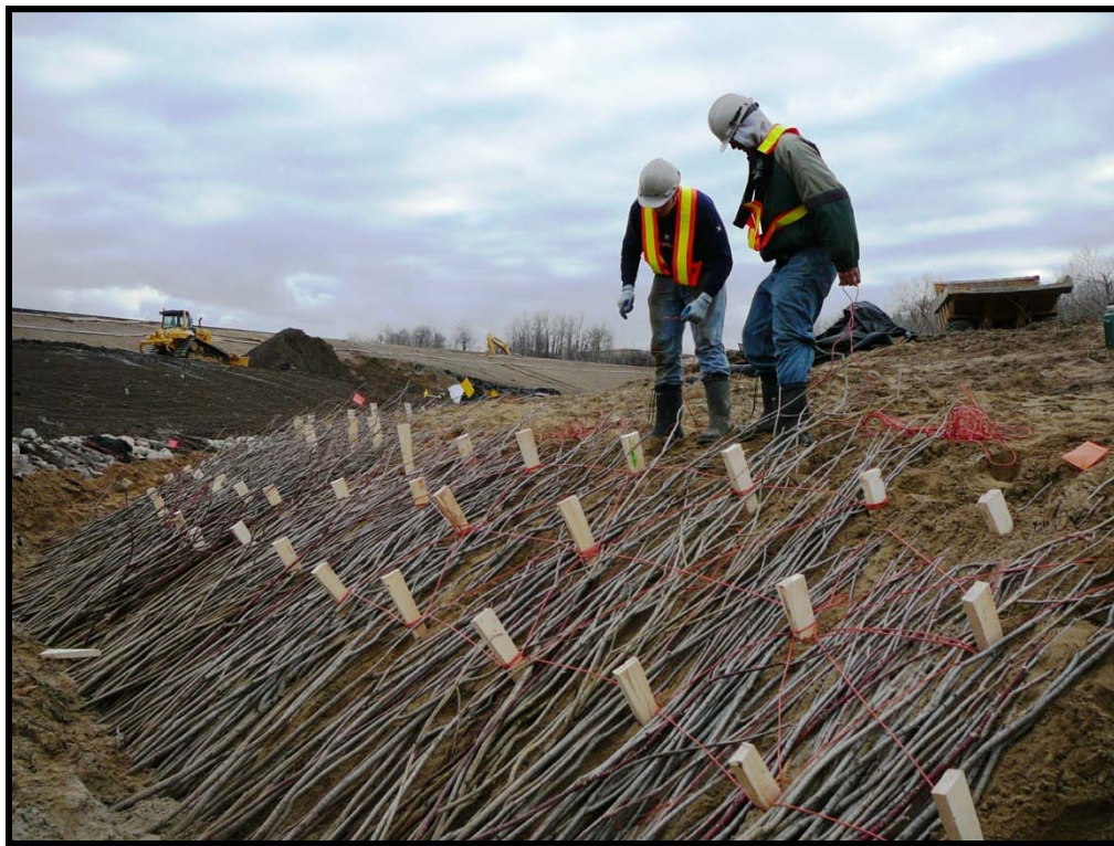
FIGURE 3.14-1 EXAMPLE OF BIOENGINEERING – BRUSH MATTRESS CONSTRUCTION (MHI, 2007)
