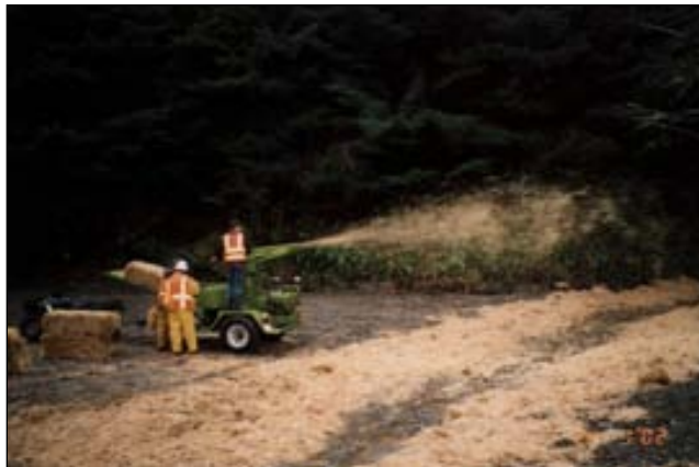
FIGURE 3.6-1 STRAW MULCH APPLICATION (NORTH AMERICAN GREEN, 2003)
