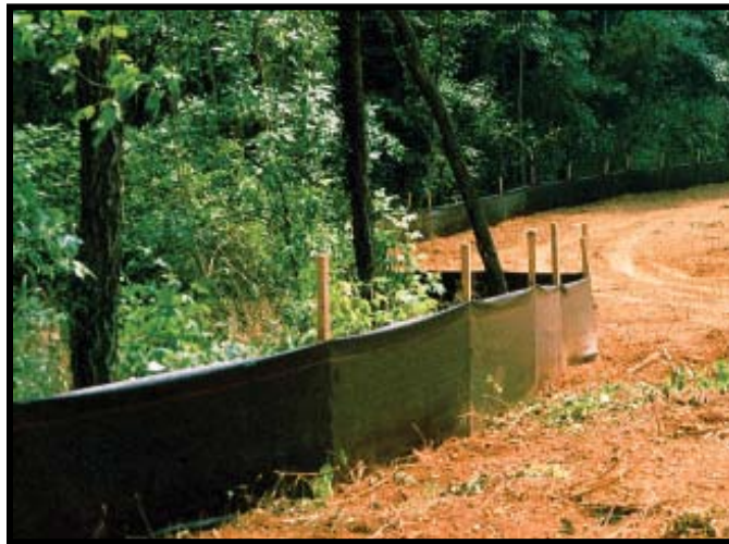
FIGURE 3.8-1 TYPICAL SILT FENCE INSTALLATION (NILEX, 2010)
