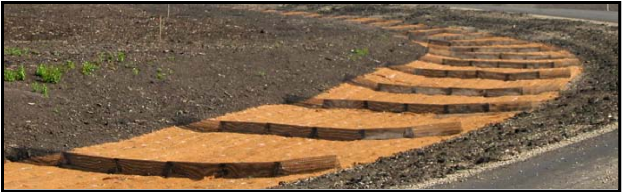
FIGURE 3.9-1 CHECK DAMS CONSTRUCTED USING GEORIDGES (NILEX, 2010)
