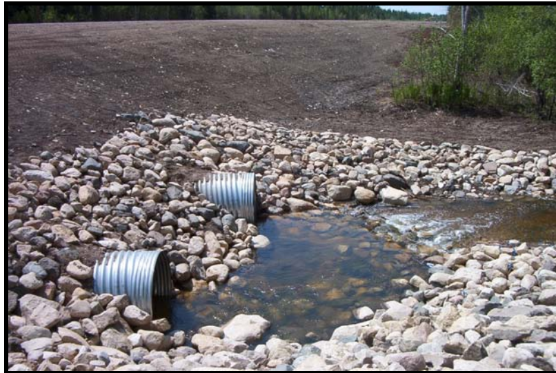
FIGURE 3.12-1 TYPICAL CULVERT RIP RAP INSTALLATION (MHI, 2007)
