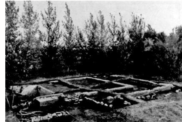
Foundations after excavation
