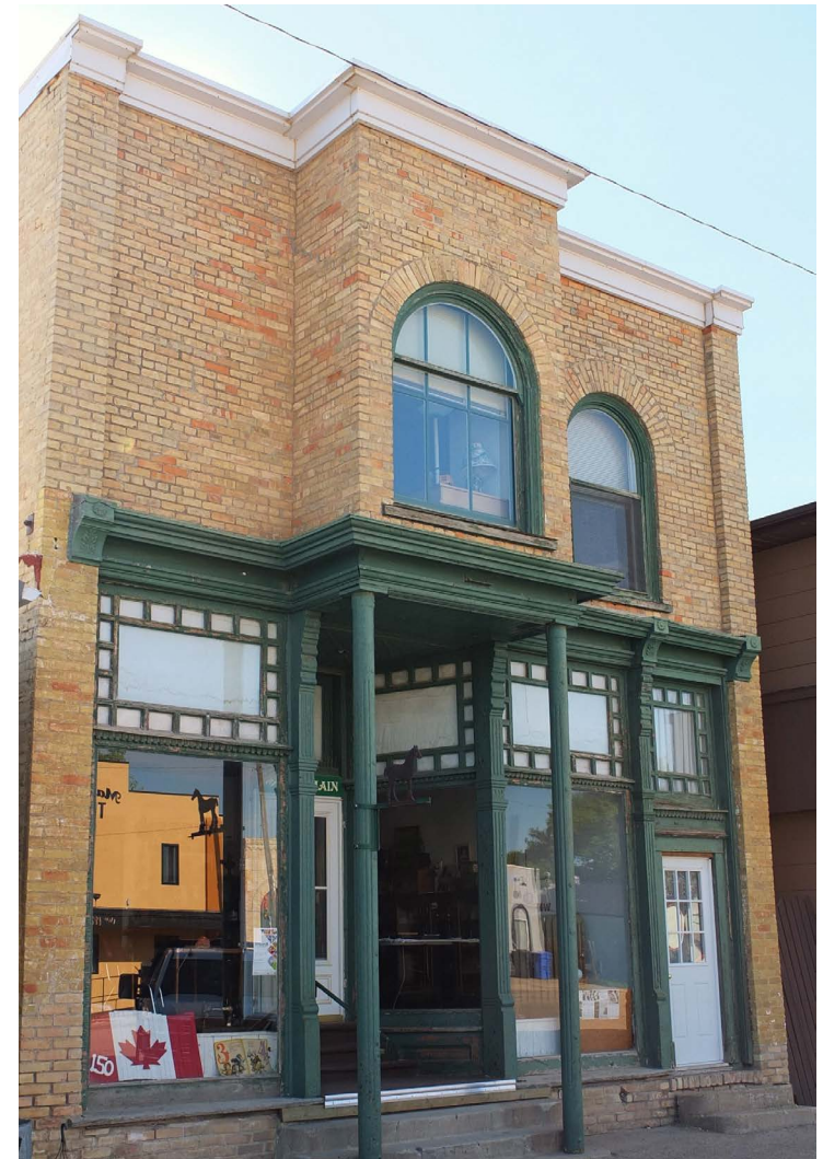
The adaptive reuse of the Pharmacy Building in Arcola involved rehabilitation of the deteriorated brick walls and foundation, as well as preservation of the relatively intact windows and façade elements.
