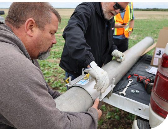
Installation of electromagnetic flow meters
