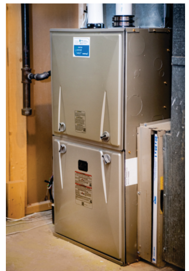
New high-efficiency furnace installation as part of the Heating Affordability Program (HAP)
