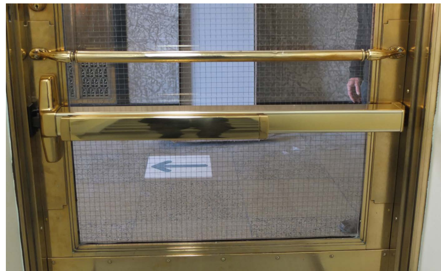
Installing a modern push bar matching the colour and finish of this historic door met code for safe egress.
